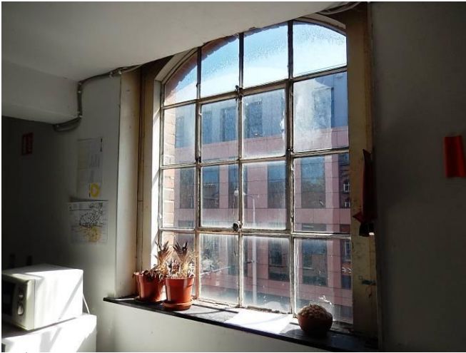
2 nd floor, view of original metal window.
