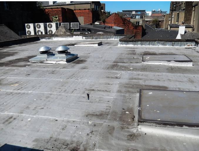
View of flat roof to northern end of rear extension
