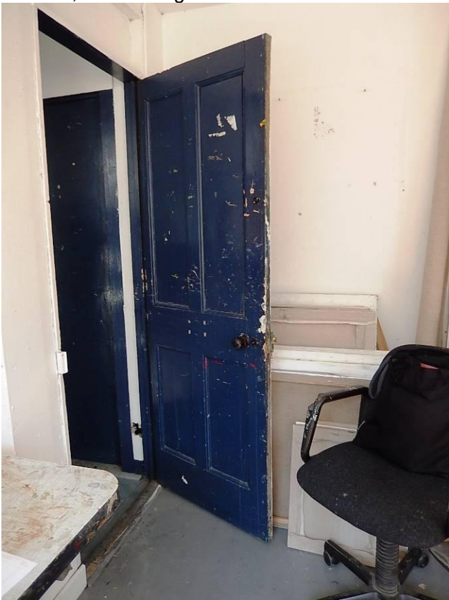
2 nd floor with original door intact.
