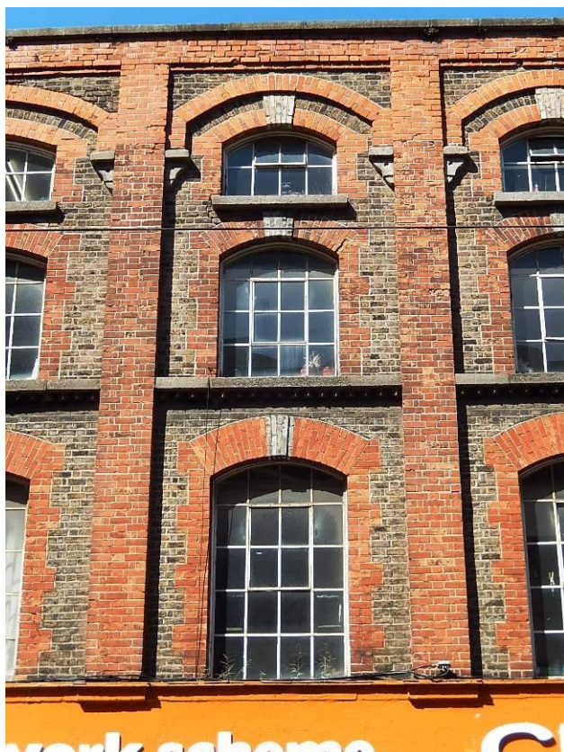
Polychromatic brickwork, keystone details and surviving upper floor windows.
