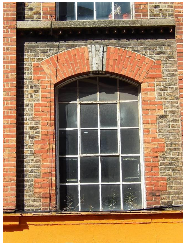
Surviving upper floor window with metal window still intact.
