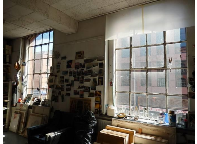
1 st floor, street fronted studio with original metal windows.
