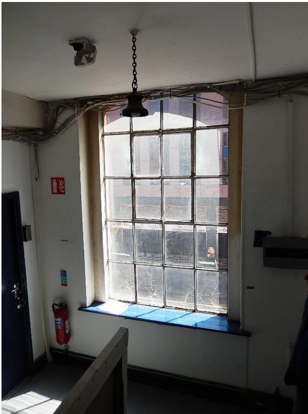
1 st floor landing with original metal window.
